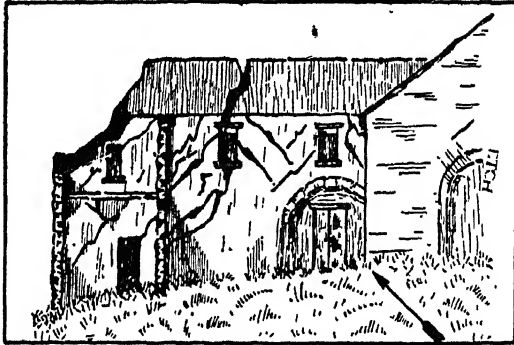
FIG. 336.—Sketch showing a house rent by earthquake shocks. The arrow shows the direction from which the earthquake wave emerged. ( Redrawn from Mallet. )
